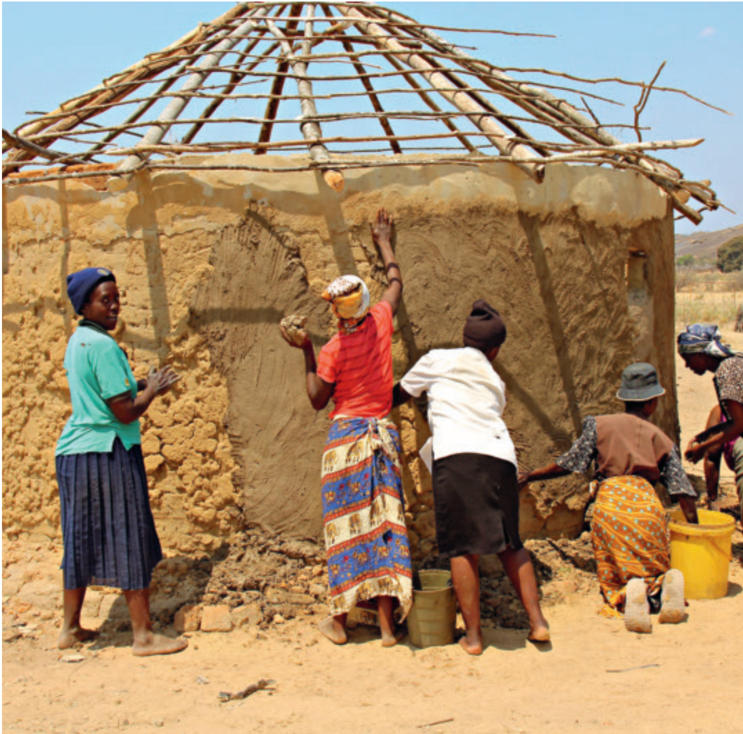
The community of Lukhanyiso building a new structure for the preschool.
